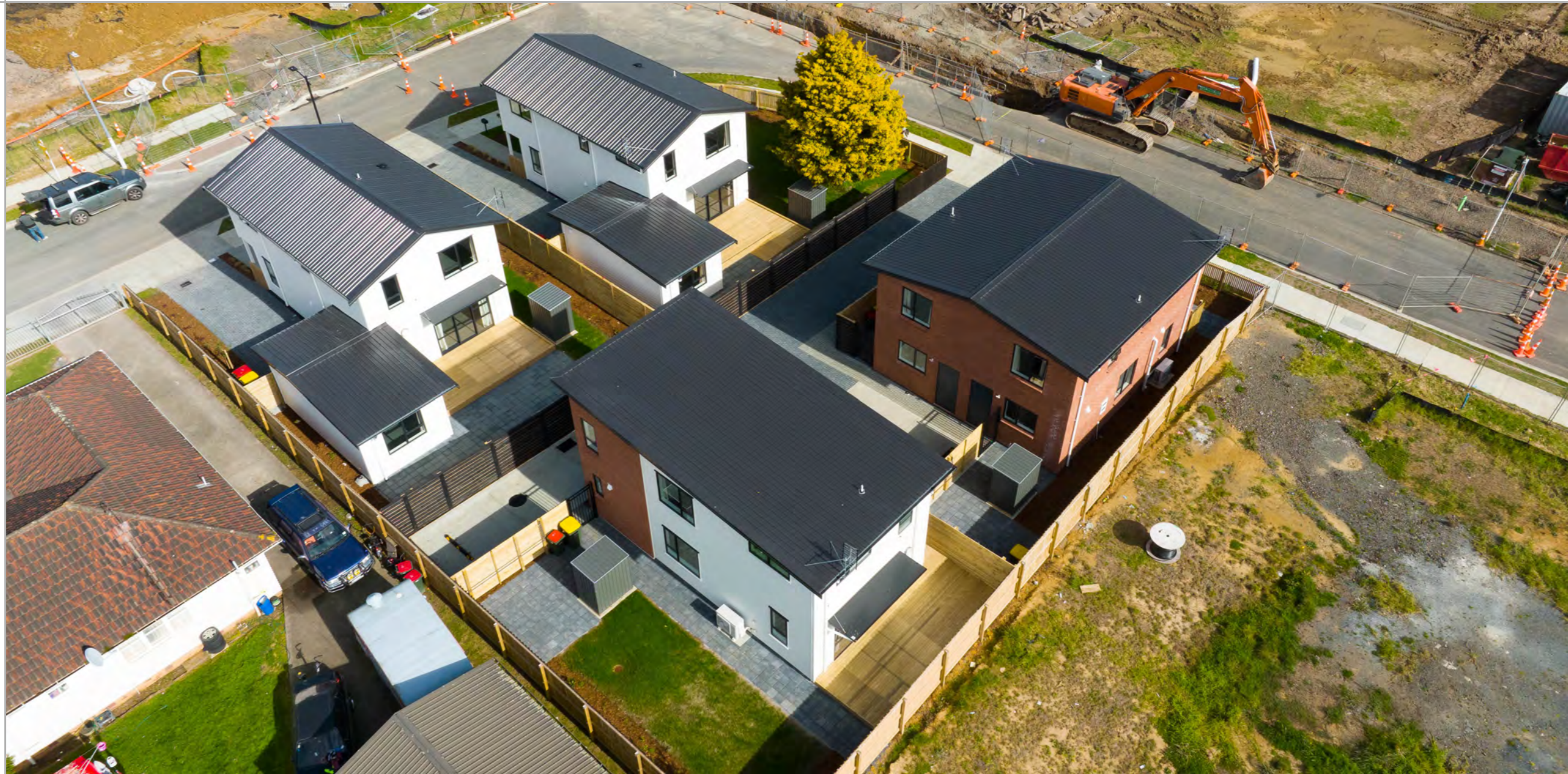
Aorere New housing at Mayflower Close - development progressing.
