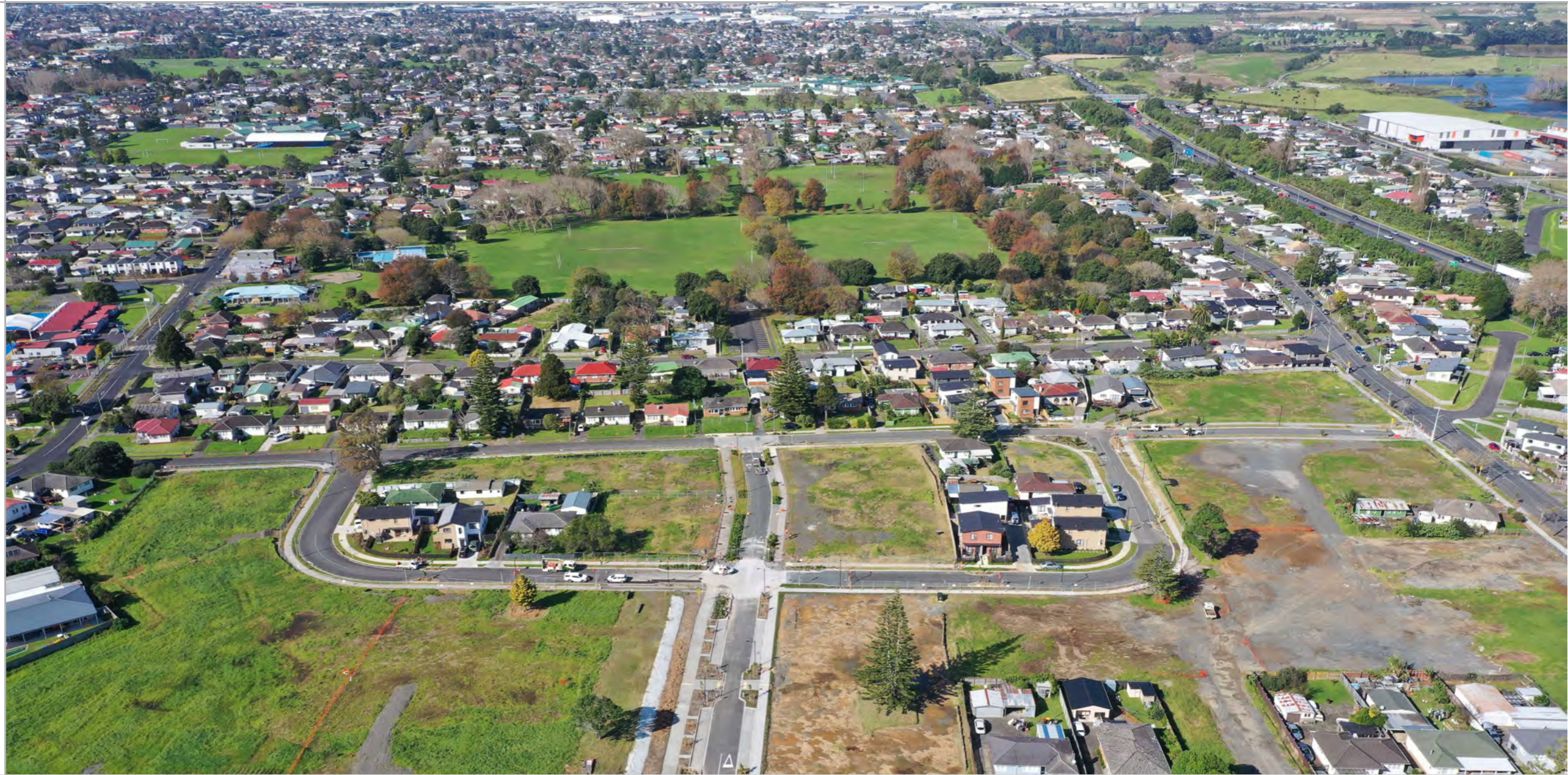
Aorere looking south along Paneke Street - the new park edge street and connection. Development under way.
