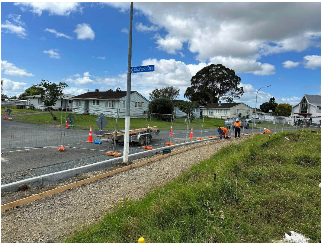
Photograph 6: Construction of sideway subgrade along Winthrop Way
