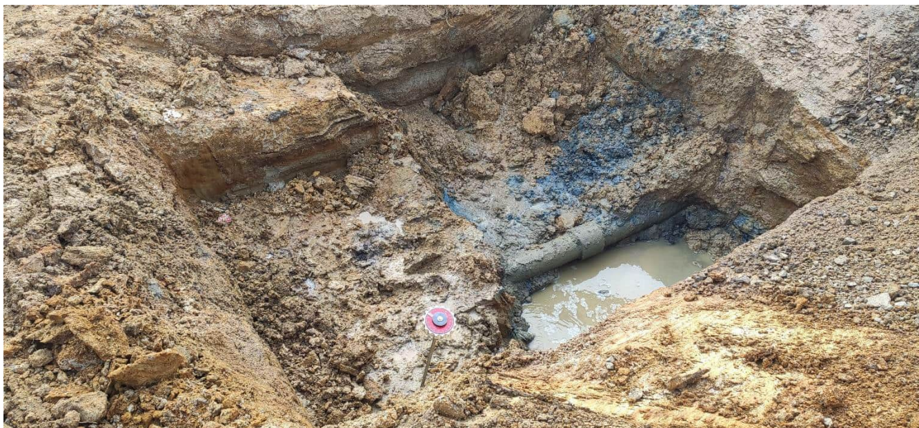
Photograph 1: Existing wastewater pipe visible running through centre of excavation. Blue grey alluvium at the base.
