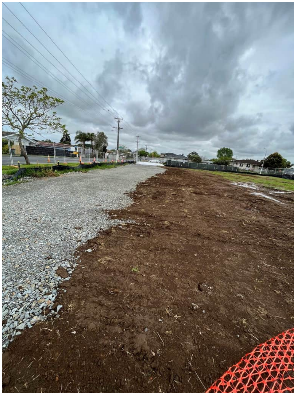
Photograph 2: 3 m wide Granular backfill strip on Superlot boundary with Henwood Road.
